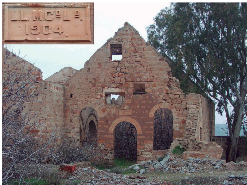
Figure 10. The engine house for the new 1904 winding engine still survives. The insert (top left) shows an inscription located over the central doorway commemorating its construction. (Author)
