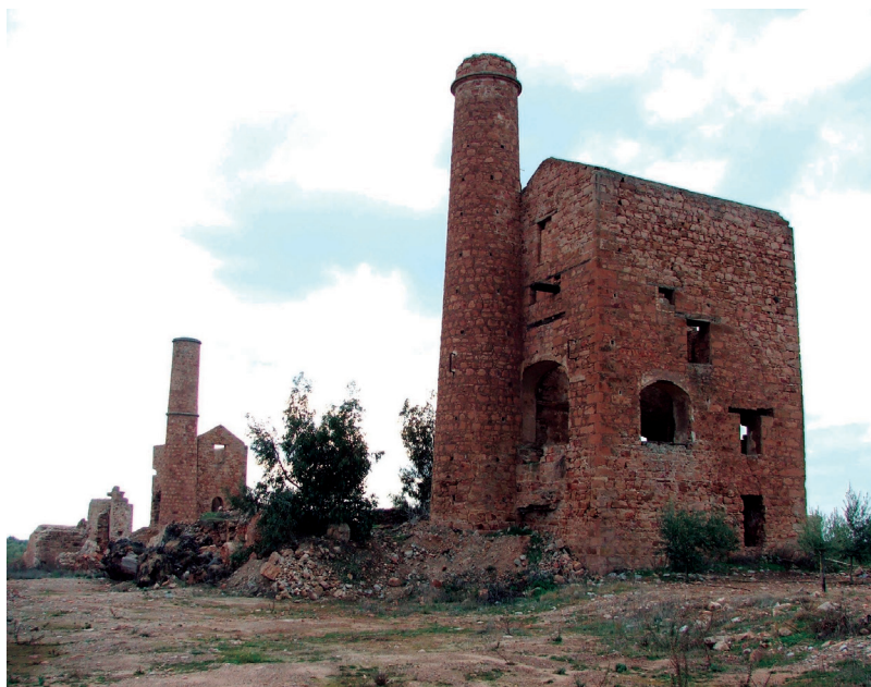
Figure 12. Pozo Ancho 2012. The two engine houses for the pumping engine (foreground) and whim engine dominate the site of San Thomas shaft. (Author)
