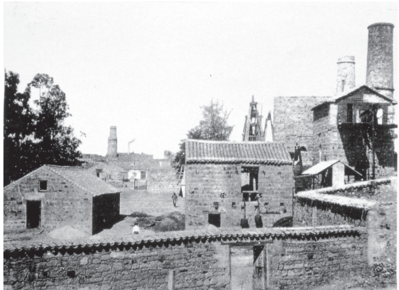
Figure 6. Pozo Ancho mine, probably in the early 20th century. The head-frame and engine house at San Thomas shaft can be seen in the middle distance. The building on the right contained the whim engine that also worked the ore-crusher (middle building in the foreground). (Proyecto Colectivo Arrayanes)
